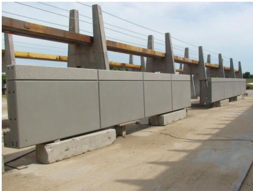
a.) Sand-Blasted Side of Spandrel Beam Storage
