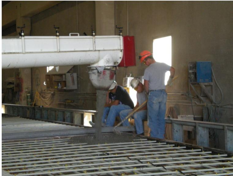
Figure 4.6. Concrete Placement for Deck Panels.
