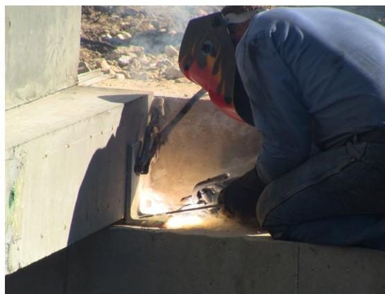
Figure 4.11. HSC Beam Welded to Abutment.
