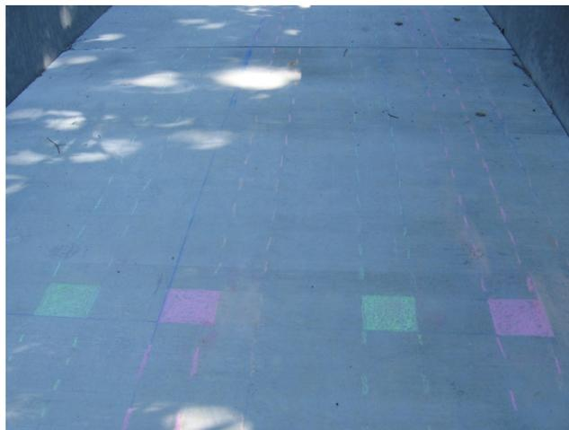
Figure 11.2. Example Fork Lift Load Path Markings.
