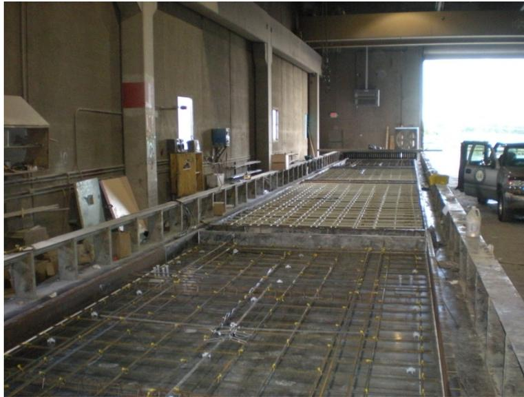
Figure 4.5. Formwork, Steel, & GFRP for the Deck Panels.
