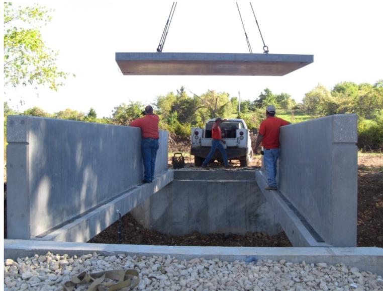
Figure 4.14. HS-SCC Deck Panel Erection.
